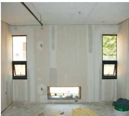
Drywall work in one of the rooms
